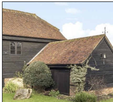
Timber framed barn
